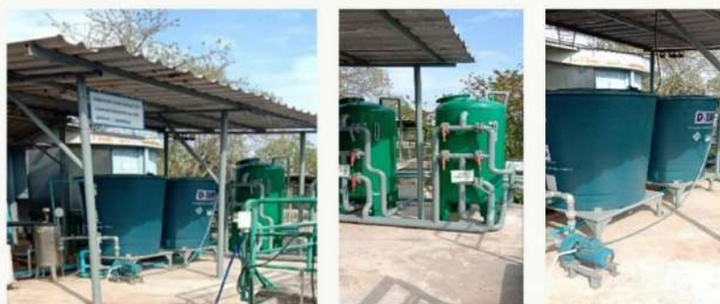
Installation of water filtration tanks for water reuse
