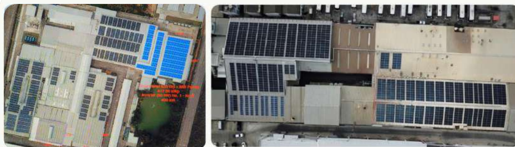
Solar panel installation on a roof
