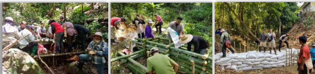
Constructing check dams in each village.
