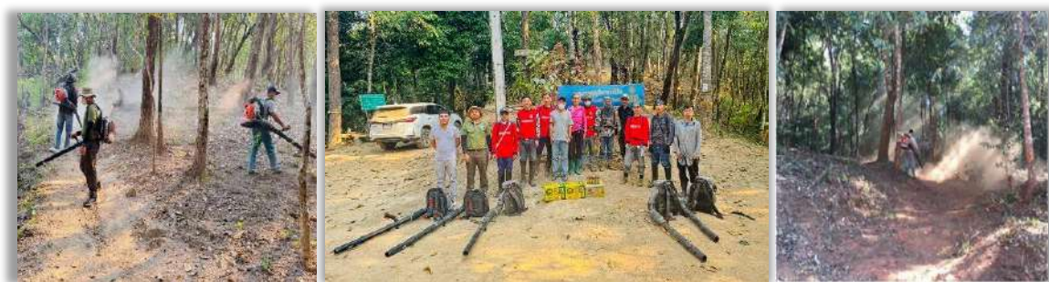
The project: Construction of firebreaks and provision of support supplies to workers.
